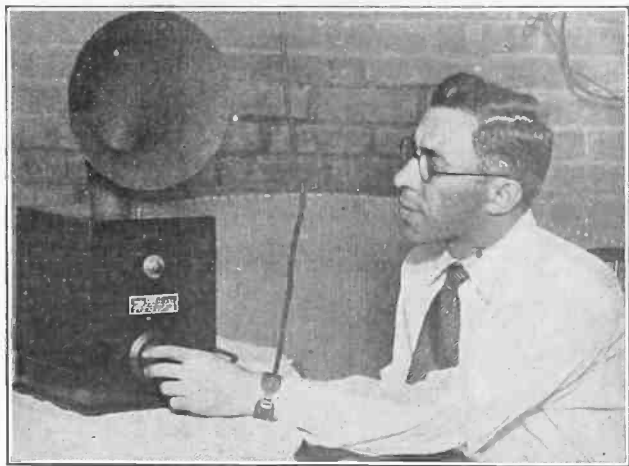
CRYSTALS as radio-frequency amplifiers are being tested by the Bureau of Standards in Washington, D. C. H. DeGroot is shown engaged in research work. At left is the quartz oscillator, next the Heterodyne and at right the wavemeter to be calibrated. The arrangement is used for frequency standardization. (Henry Miller).
