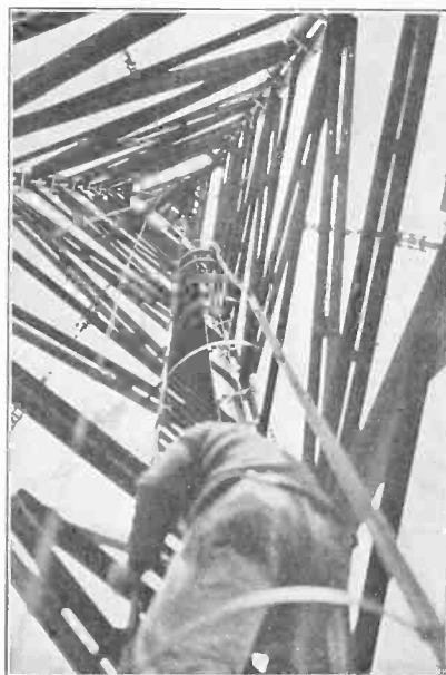
(Fotograms) ANOTHER view of one of the supporting towers of the huge aerial system at the power Naval wireless station at Sayville, N. Y. The photographed climbed up the middle of one of the towers to take this photograph. At the top, which is 480 feet above ground, the towers sway in the wind.
