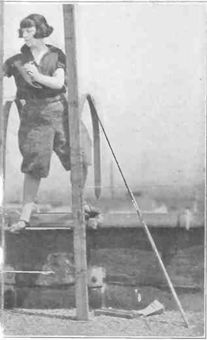
pole at least seven feet over the roof. The first thing to be done is to see that the end of the aerial wire does not come down to the ground, and that there are no kinks or knots in it. Keep it clear of surrounding objects as possible.
