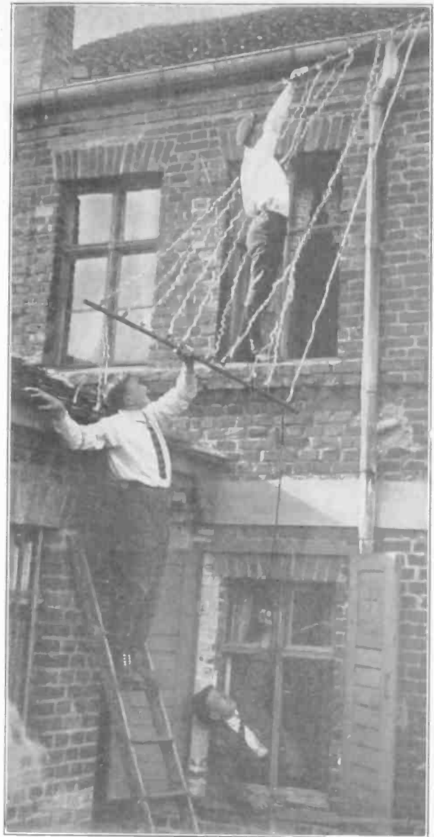
(Keystone) FIG. 7.—This is the type of antenna in vogue before broadcasting began. It consists of a number of wires in parallel, fastened to a spreader at each end by an insulator. The greater number of insulators in parallel, the lesser the resistance. Hence, use a single wire.
