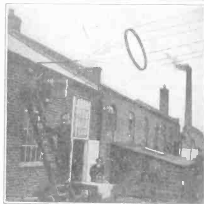
THE NEW high-wave experimental station of the British Broadcasting Co., call letters 5XX, uses the above cage aerial. The station, at Chelmsford, tried to transmit to America during the tests.
