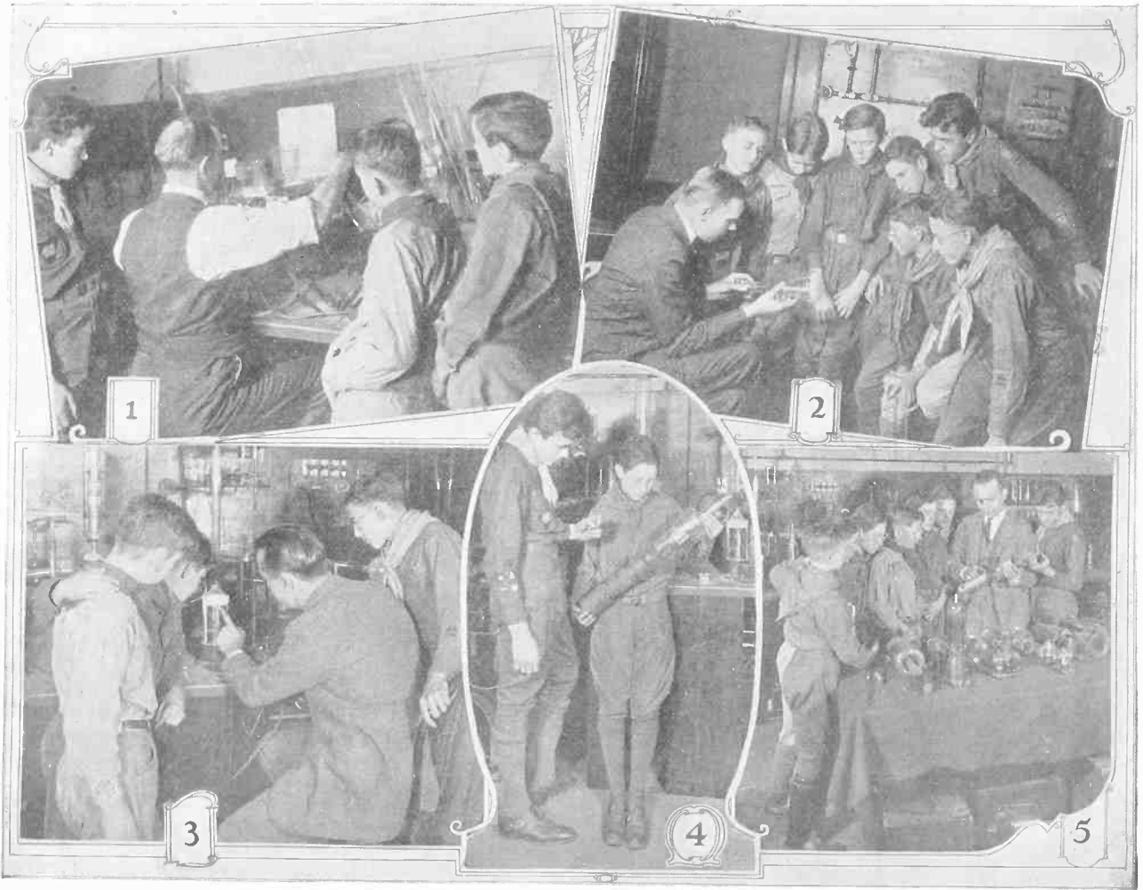
SCOUTS of Brooklyn and Queens inspected the Bell system laboratories. (1) First step in manufacture of 10,000 watt tube; (2) J. B. Johnson, inventor, demonstrating; (3) measuring strength of heated wire in vacuum; (4) two extremes of tubes; (5) finished products.
