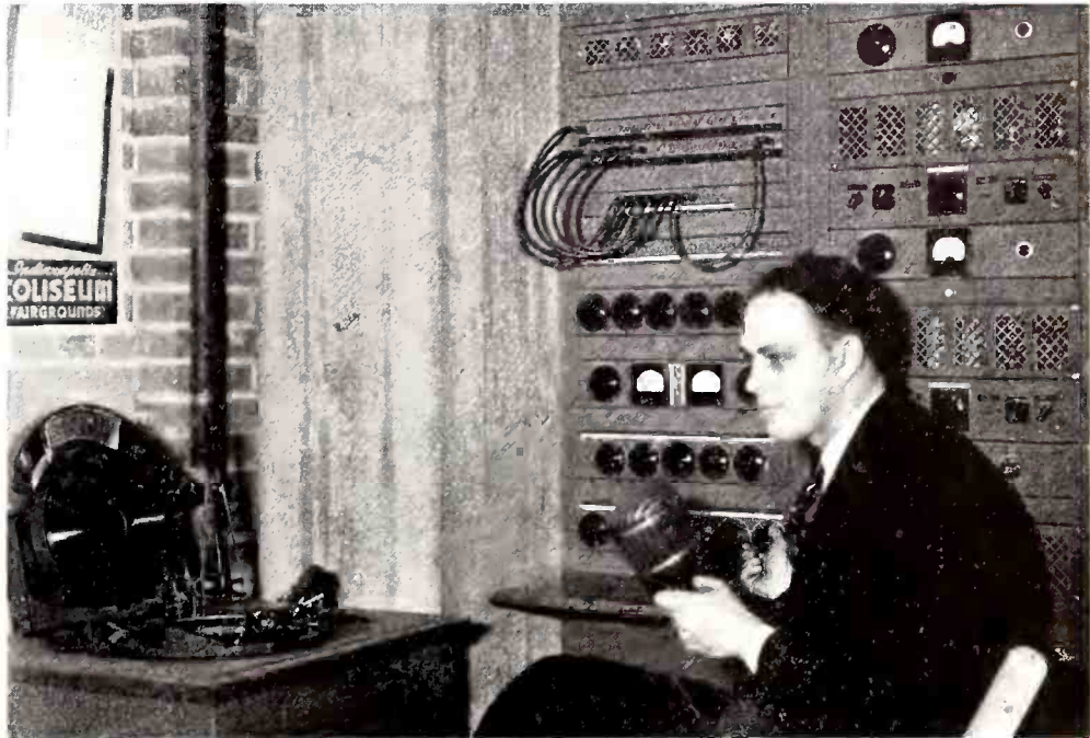
Here is the operating position of the Coliseum PA system. Rack-mounted Operadio equipment has patching and gain control panels on left, amplifiers on right. Portable record changer shown in lower left corner.
