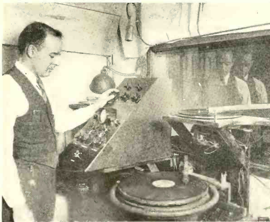
Cathode-ray oscillograph monitoring is employed in W2XR's control room in place of the sluggish power-level meter. Two pairs of turntables allow for the reproduction of all types of recordings including high fidelity.
