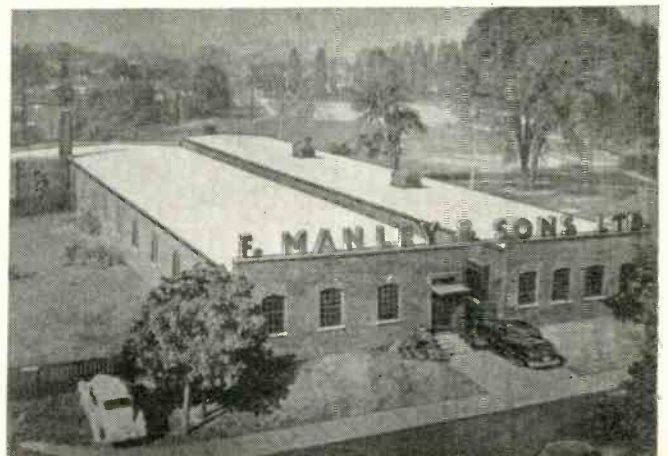
Shown above is a photograph of the fine new building of F. Manley & Sons Ltd., located at 198-200 Laughton Ave., in Toronto.
