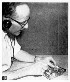
Listening in on an antenna trimmer adjustment, and of several steps in aligning the set.
