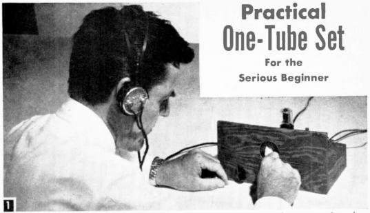
Unhampered by a tiny cabinet, the novice can easily put together this basic circuit in four stages, testing as he goes along to "see" how a radio works. Scrap wood panel and base afford room to rearrange or add parts.
