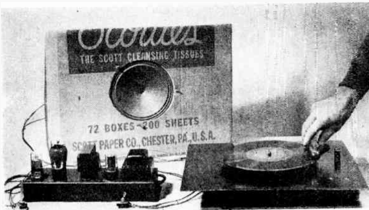
Fig. 7. The speaker is mounted in corrugated carton. The motor and the amplifier units are then fitted together in this temporary set-up.
