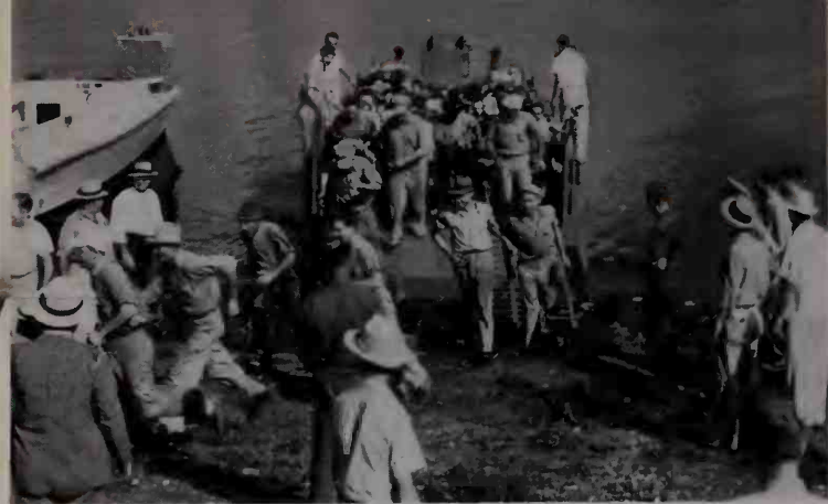
Left . . . One of the 45-foot HIGGINS' built, welded steel, twin screw, diesel powered tank carriers takes a labor battalion for a boat ride. Off the boat came 187 men.
