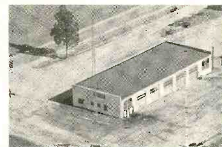
Fig. 1—Salem County Road Dept. installation. Note the antenna.
