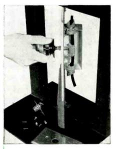
Fig. 6—Typical hole cutting procedure in tapping coaxial line.
