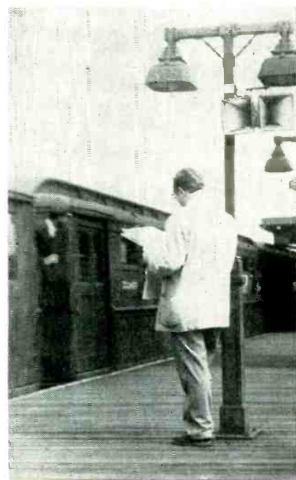
Fig. 3—Paging systems are used increasingly on subway surface lines.
