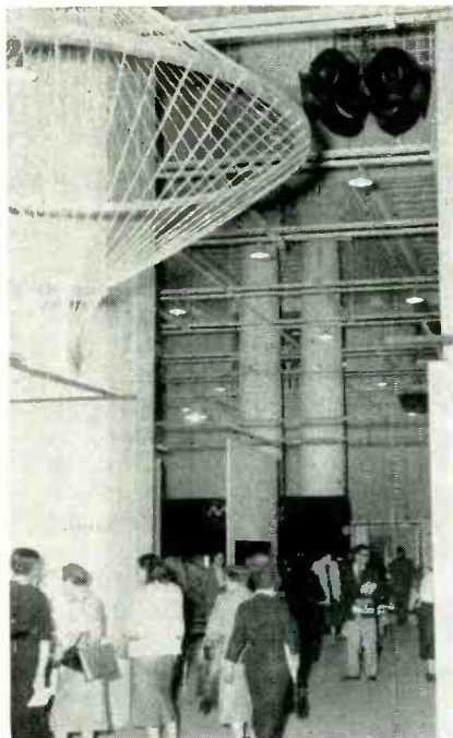
Fig. 2—Cluster of p.a. speakers set up for announcements and music.
