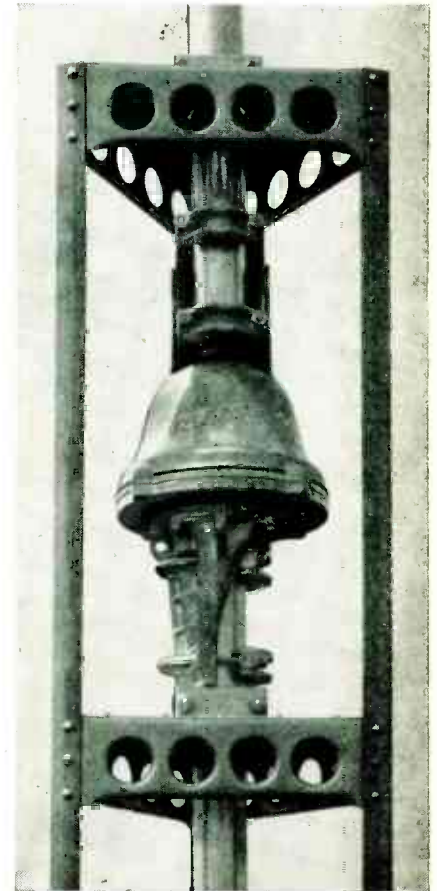
Fig. 9. Tele-Rotor mounted inside tower or superstructure.
