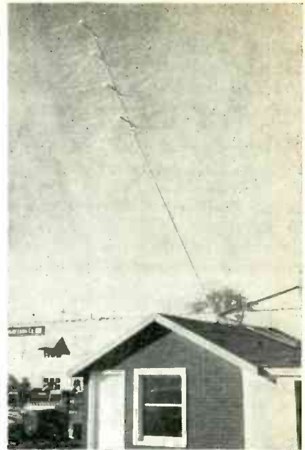
Fig. 4. Mast almost completely raised vertically.
