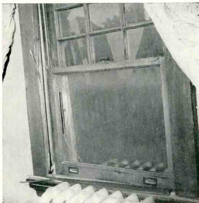
Fig. 3 (below). Interior view of the top window showing the extent of damage done at this point. The violence of the shock splintered the inside framework, broke the window pane, and shattered the plaster on the wall.
