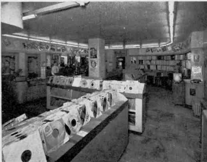
Interior of the Jackson Blvd store
