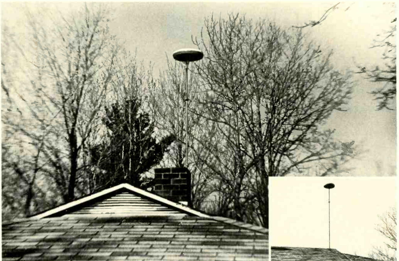
RCA's Model 5MS440 Mini-State Antenna System mounted 10 ft above the roof of your editor's home. Note the trees, which can be a source of reflected TV signals.
