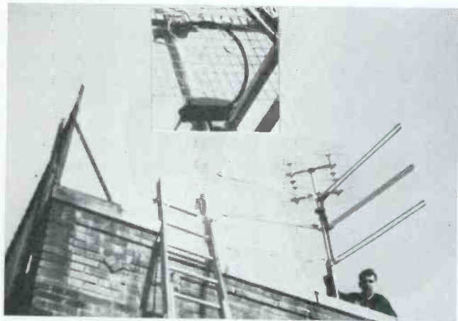
One of the more elaborate UHF/VHF arrays used in the New York test. Note the cross-over network which permits the use of one transmission line.
