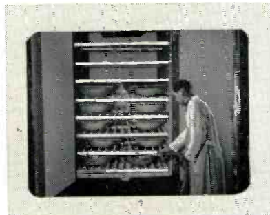
Drying ovens remove moisture from phosphor
