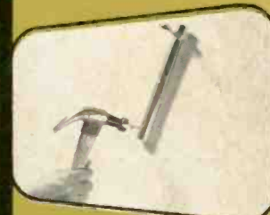
Nail up mounting bracket.
