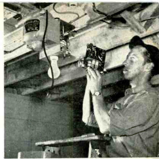
Fig. 5: Installer about to insert radio receiver in housing containing motor and electrical operator controls.
