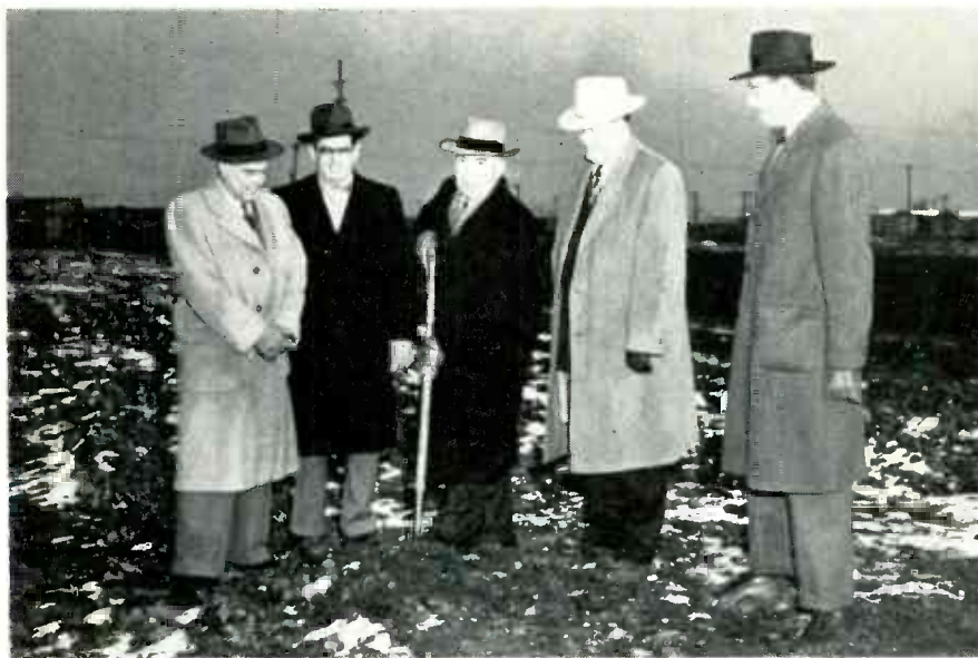
The weatherman failed to dampen the spirits of this group of Motorola, Inc. officials who dug the first shovel-fuls of dirt at the Chicago site of the firm's $3,000,000 TV plant scheduled for completion by October. Shown left to right are Edward R. Taylor and Walter Scott, Motorola vice-presidents; Paul V. Galvin, company president; William J. McNerney, mayor of Franklin Park; and John Cromelin, architect. The giant plant requires its own water system.
