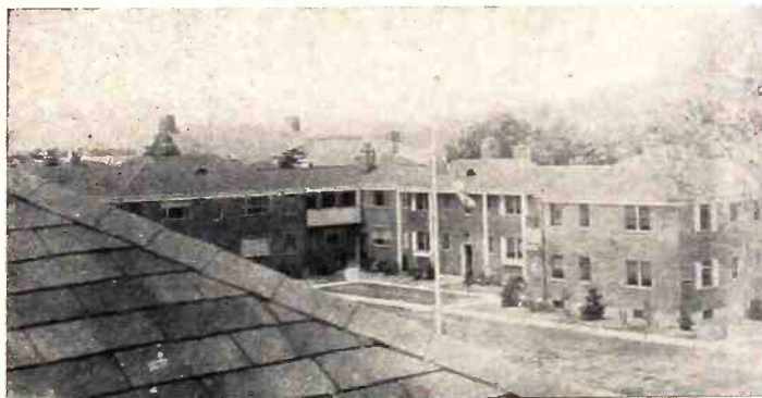
This is a cross-section of the Port Washington, Long Island, project at which the master installation was made using the WARREN CORONET .
