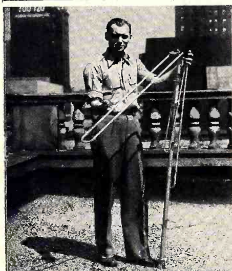
Dick Moss, television engineer, flicks up dipole in assembly operation of Ward Minute Man antennas. (Model TV-46).
