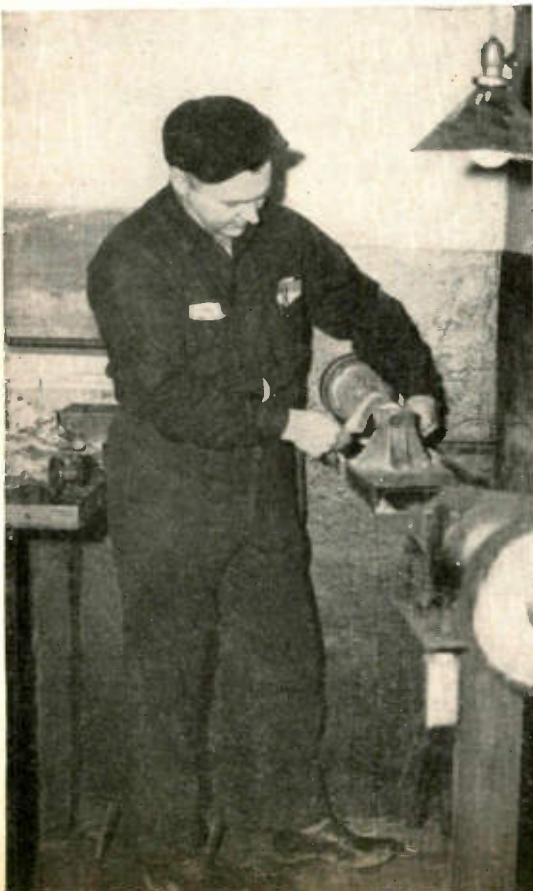
Cut down a washer wringer roller (rubber), and sand it to smoothness? Sure, as this repairman is doing in the corner in this photograph.
