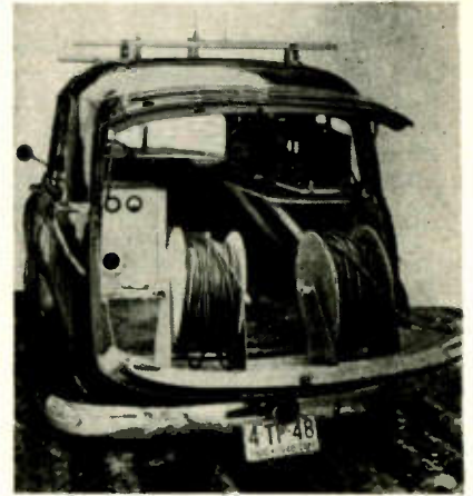
Ward mobile testing laboratory used to check firm's new television aerials in the field.
