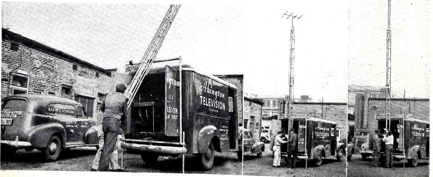
Below: Lowering the tower into position from its resting place on the roof of the truck. Right: tower in position at a height of 25 feet.
