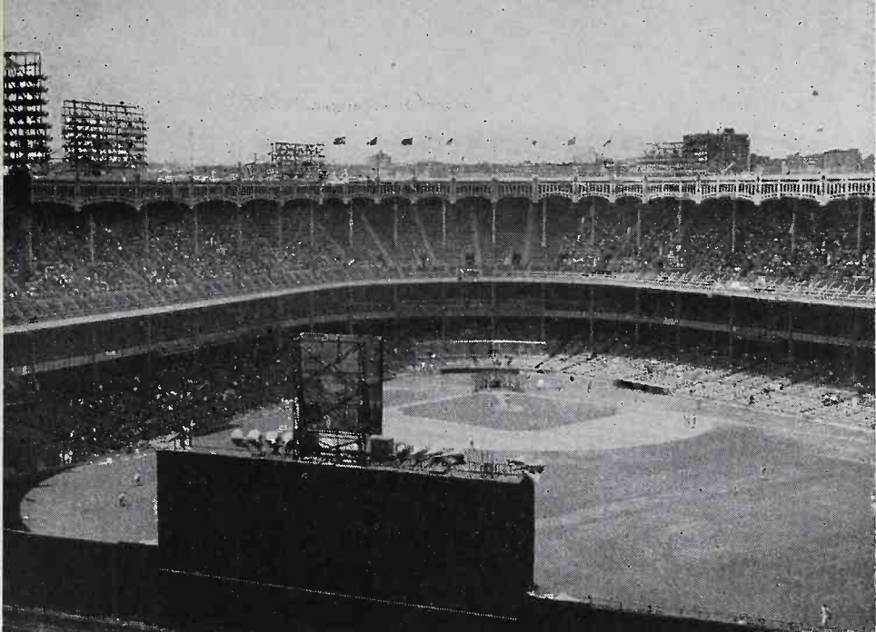
"Over the shoulder" of the loudspeaker battery at the Yankee Stadium. Eight 6' trumpets are aimed to cover 120°, with two RCA "twin-power" cube speakers added in a concentration toward the front to cover the relatively longer distance to the stands. The six inside trumpets carry two units each. For bleacher coverage, four 5½' re-entrant horns are used.
