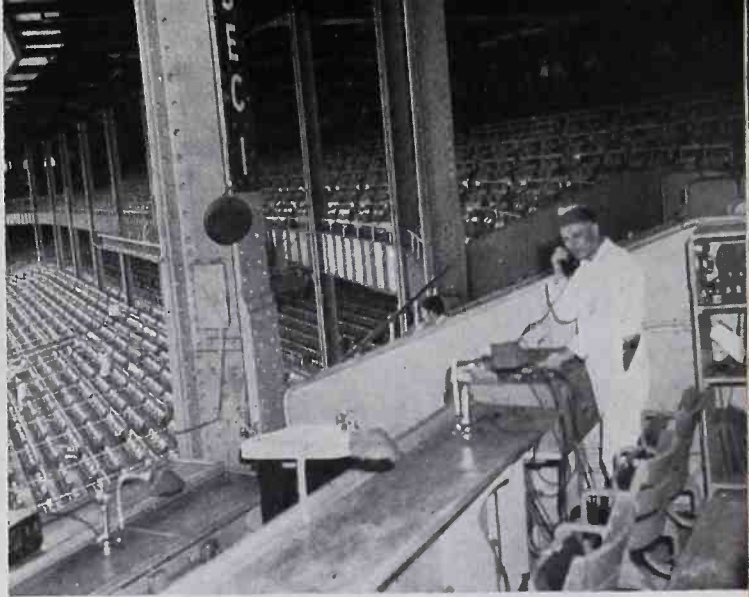
Microphones are used on the field for special events, run on cables from terminal boxes in the Yankee dugout, terminating at the operator's control booth, seen at the right. Scorer's position, next to water cooler, has intercom and mike, while at operator's left is the announcer's mike. Behind operator are booster, 50W club amplifier and 25W scorer amplifier, records and supplies.
