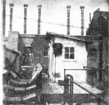
Cleaned samples are weighed in the tare house (close-up) and the percentage of weight loss microphoned back to the weigh house, where calculations show the net. The plant pays on this basis. Formerly, truckdrivers passed weight slips to the tare house at the end of a long stick
