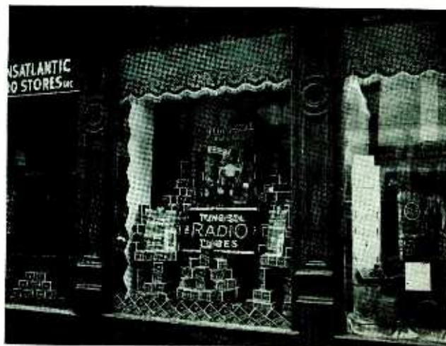
Section of the imposing spread of Trans Atlantic's show windows facing Cortlandt and Washington Streets
