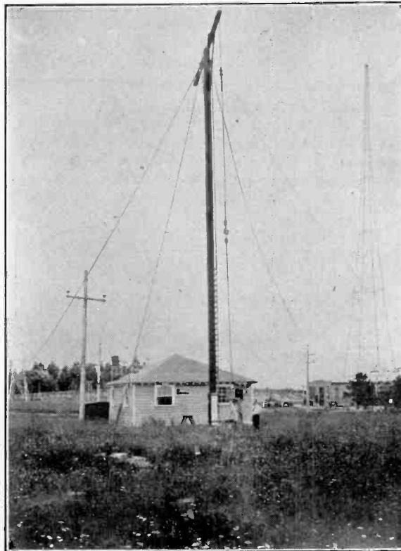
Fig. 5. Wooden Pole is Used as Tower for High-Speed Aerial
