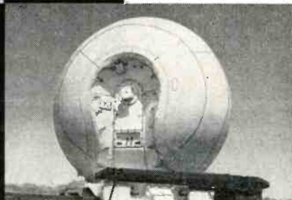
Two tracking-radar antennas, housed in radomes, take over. One feeds target azimuth, elevation, range data to computers; other tracks Hercules.
