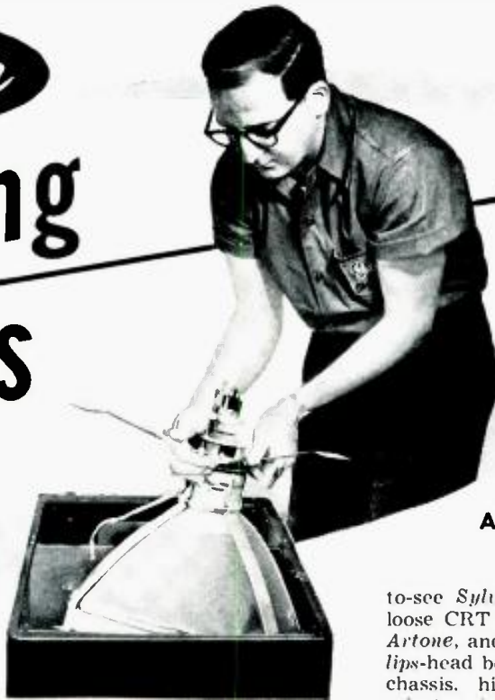
Fig. 1. Unless this set was laid face down, it was an almost impossible job to remove the CRT from the cabinet, unless you happened to have three hands.
