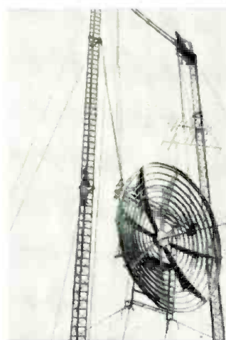
rigidly-braced steel structure. Reflecting wire mesh covers its surface.
