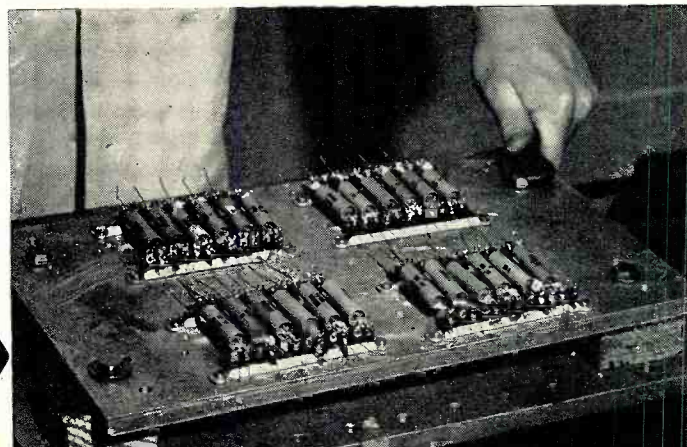
Oil-filled capacitors are subject to vacuum under elevated temperatures, then are individually examined to insure complete hermetic seal.
