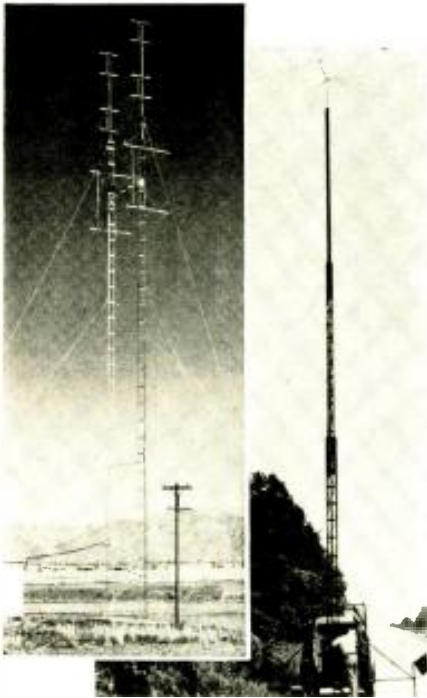
Left, antenna towers of the community TV system at Cuyama Valley, California. The yagi antennas pick up seven channels from Mt. Wilson, 125 miles away. Right, a typical mobile antenna tower unit for making field strength surveys to find the best antenna site for a community TV system. This tower can be handled by one man and mounts on the roof of the truck after being cranked down into the bottom section.
