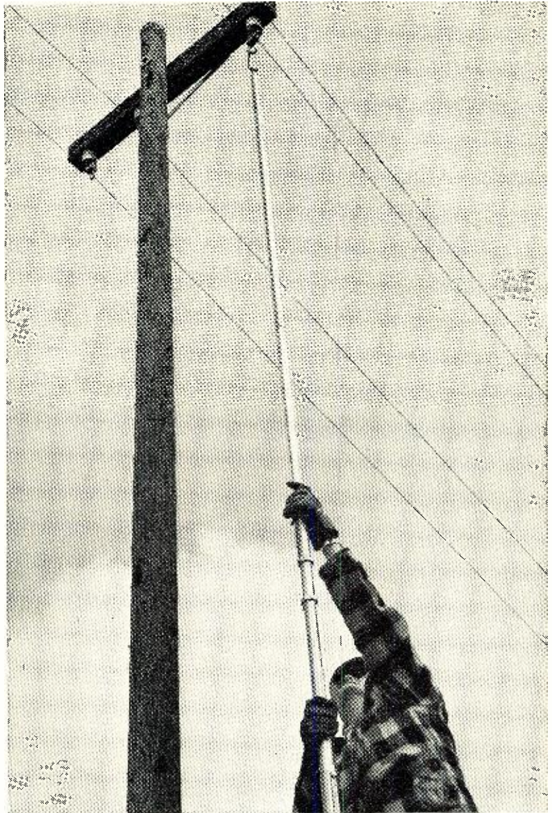
Fastening wires with new tool.
