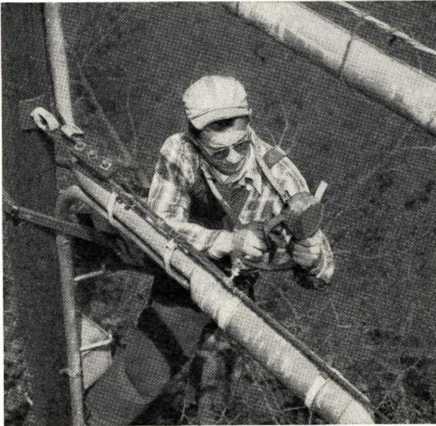
Air compressor and tank are at right. Long cylinders on rack dry air before it enters cables.
