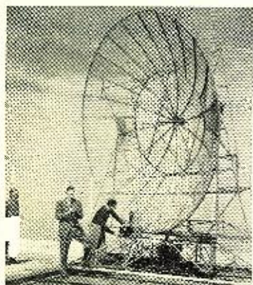
COVER PHOTO: Don Lee's 16 foot parabolic reflector (known as the "Mountain Shooter") located atop Mt. Lee, California, is believed to be TV's largest dish. (Cover photo by Mark Finley)
