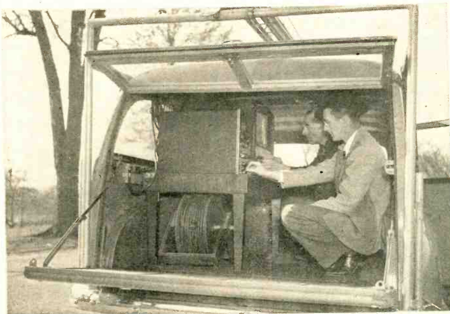
Mobile field strength test equipment unit used by Service Division of Philco Corporation shown in operation in Philadelphia.
