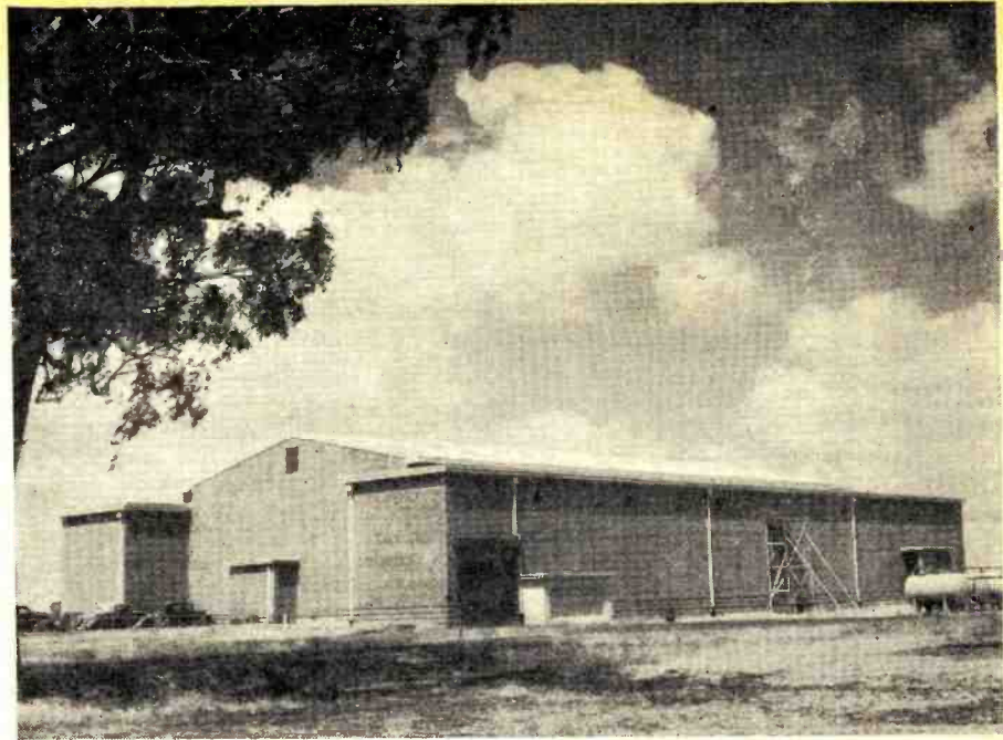
The present home of "Radio Australia." This picture shows the transmitter hall.
