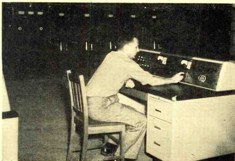
Control desk for one of the 50 kw. transmitters operated by "Radio Australia."
