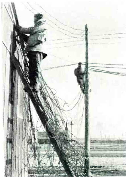
Radio students erecting wire network for PBS.
