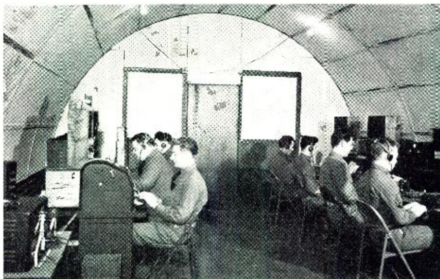
Complete equipment consists of nine super Hammarlund Super-Pro receiving and transmitting sets, one teletype printer, one code machine, and one Syphon recorder.
