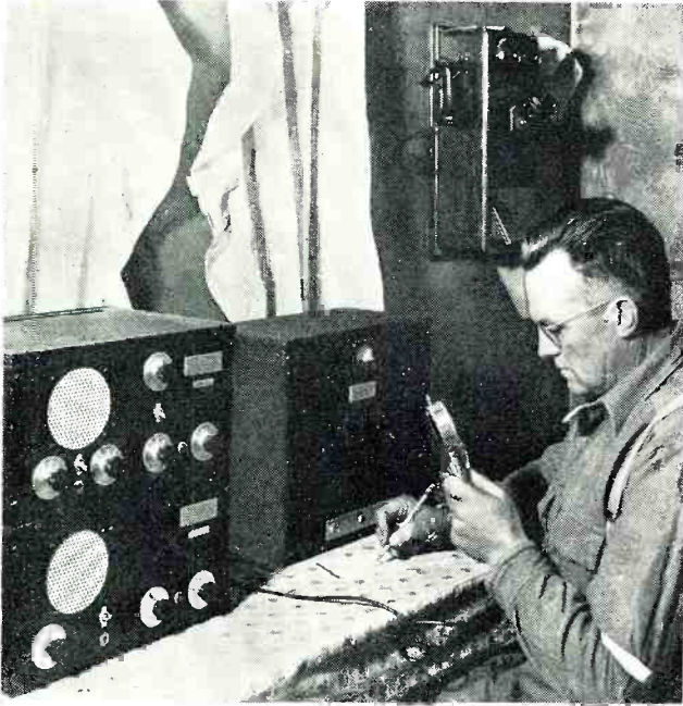
District engineer talks with plow operators giving up-to-the-minute instructions via radio.
