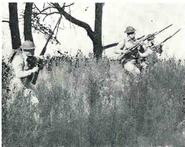
1 This advance detail is headed for a location that has been picked as a site for high-power transmitter.
