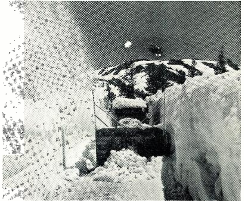
Carrying-out job of removing snow after receiving orders by radio from headquarters. Truck is completely equipped.
