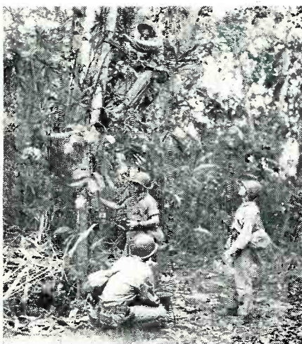
Tall coconut trees are used for telegraph poles at Guadalcanal.
