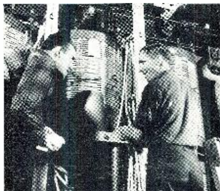
Inspecting large Power Transformer.
