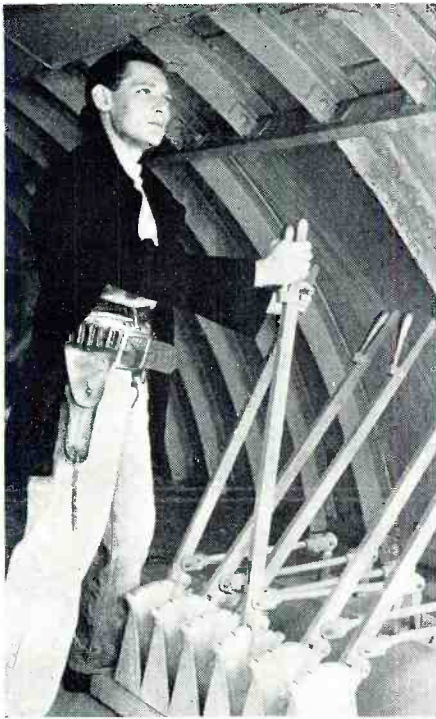
Here is an actor manipulating the submarine controls "far under sea."
