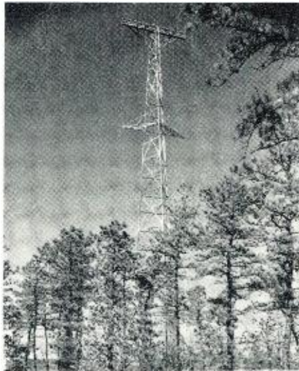
A typical 6 megacycle beam antenna.
