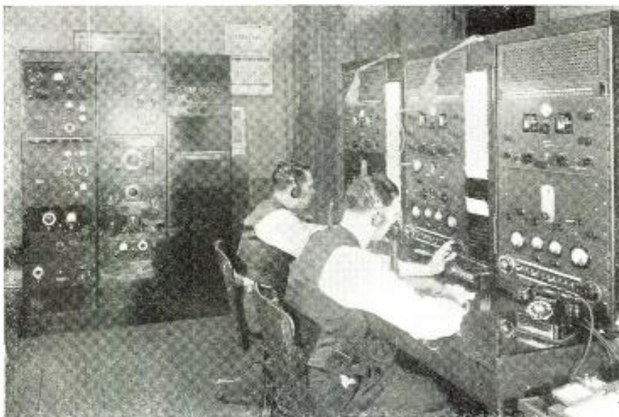
Ship radiophone calls are received here and re-routed over land wires.
