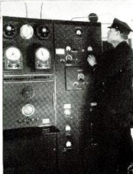
This is the remote transmitter which is used to operate the devices aboard the St. Clair . Impulses are sent automatically.
