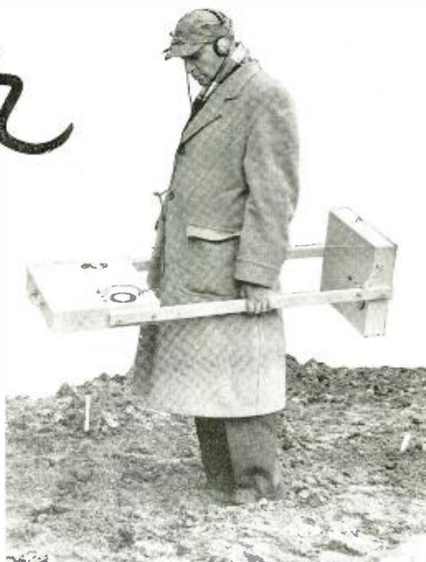
An assistant of inventor Gerhard Fisher trying out the M-Scope. If he passes any metal, meter needle deflects, and a buzz is heard.
