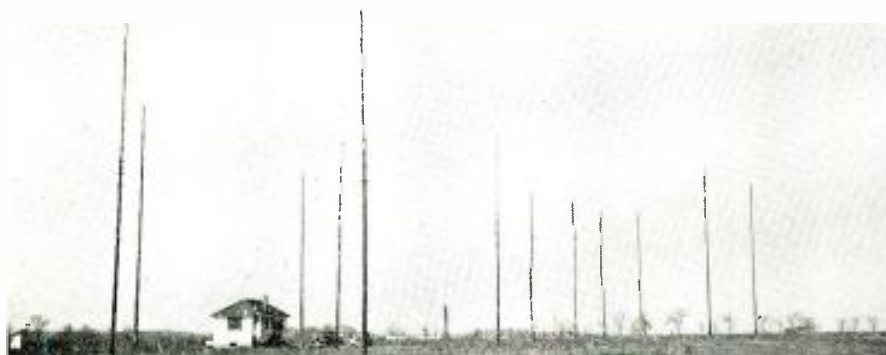
The antenna system maintained at Lorain, Ohio, for ship's radiophone. From here emanate the voice controlled transmissions which are used.
