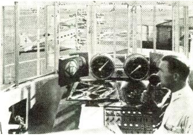
Newark, N. J., Radio Control tower is the same as most others. Ships land at the order of the "op."
