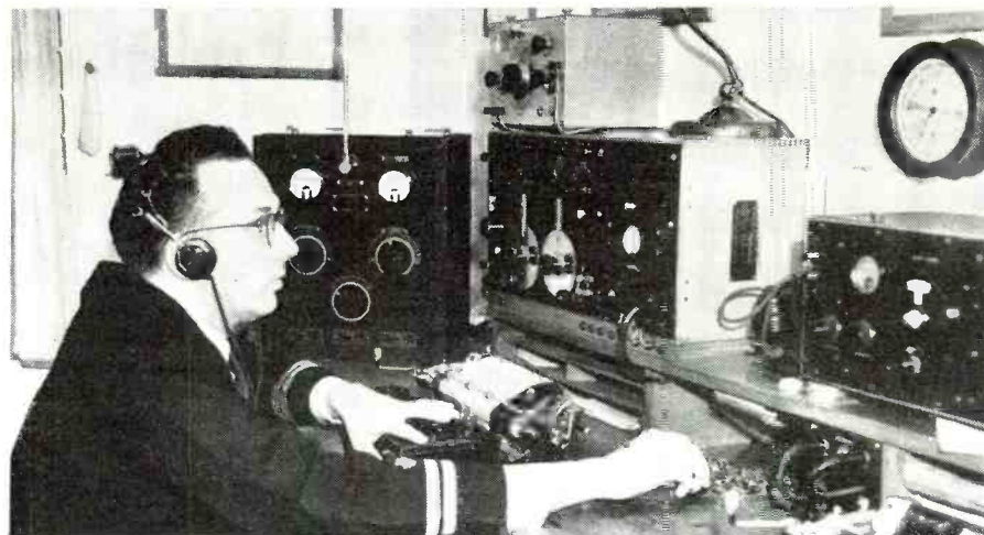
The wheel rotates the loop on the roof, and by charting the signal, Chief Officer Abbott plots the ship's position.
