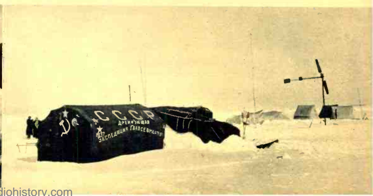
The Soviet Polar Station No. 56 on the pack ice. Note the wind-driven propeller used for charging the battery for the radio.
