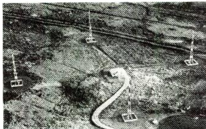
The ground layout of the "air-track" as the radio beam is known. By it pilots keep schedule accurately.
