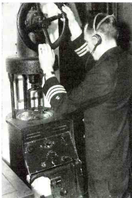
The wheel rotates the loop on the roof, and by charting the signal, Chief Officer Abbott plots the ship's position.
