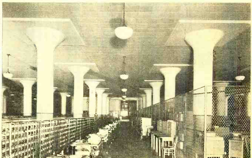
Figure 9. In this Addressograph Department of Montgomery, Ward building the ceiling is covered with Sanacoustic tile, which absorbs sounds of machines
