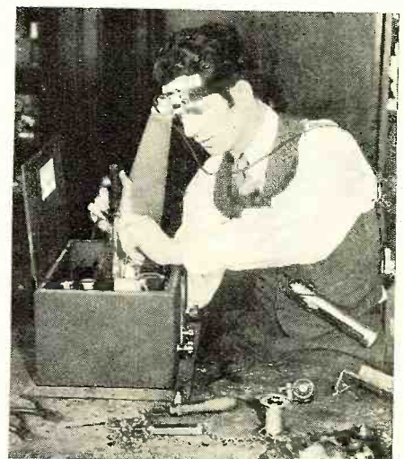
Figure 5. This handy light provides a third hand to the serviceman
