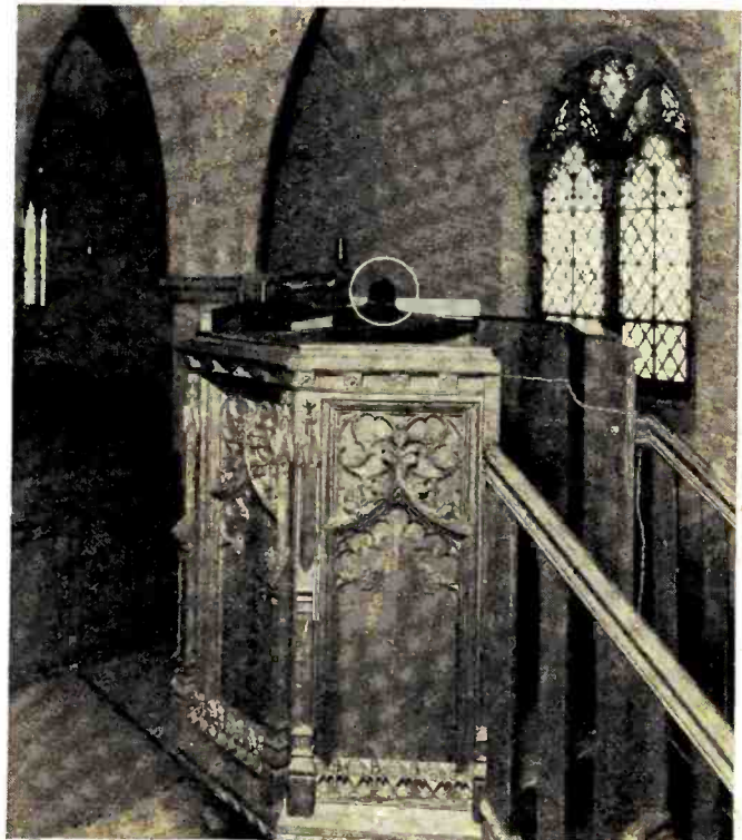
The inconspicuous microphone (in circle) may be left on the pulpit or concealed nearby. This view shows the early installation in the Reformed Church, Bronxville, N. Y. Later the microphone was placed in a concealed position fifteen feet from the pulpit
